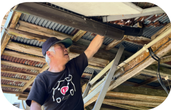
[雨樋掃除の様子]
